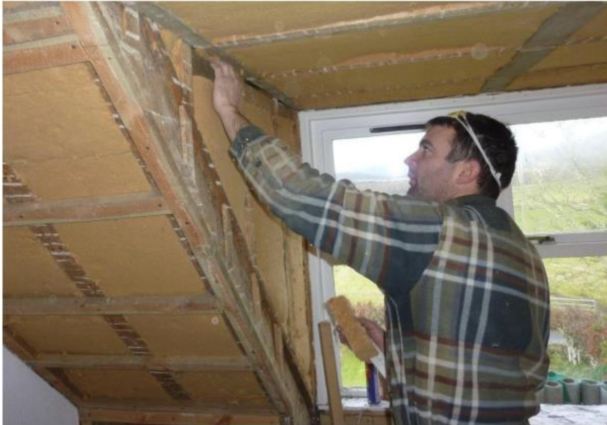
Room-in-roof insulation with wood fibre boards
