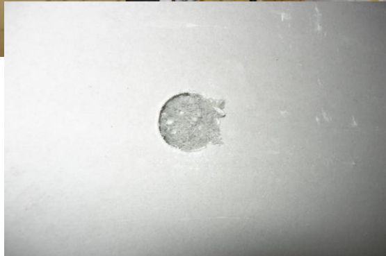
Cellulose fibre – u-Value 0.7 (48% improvement)
