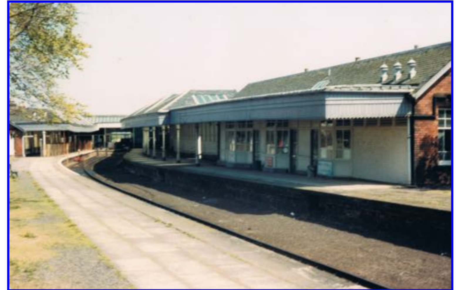
The original station buildings prior to their demolition in 1985. The second platform had been trackless for many years, and the goods yard had been closed in 1968. Photograph S. Auld
