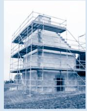
Work in progress at the Doocot in November 2006 - the scaffolding providing access for the limewashing.
